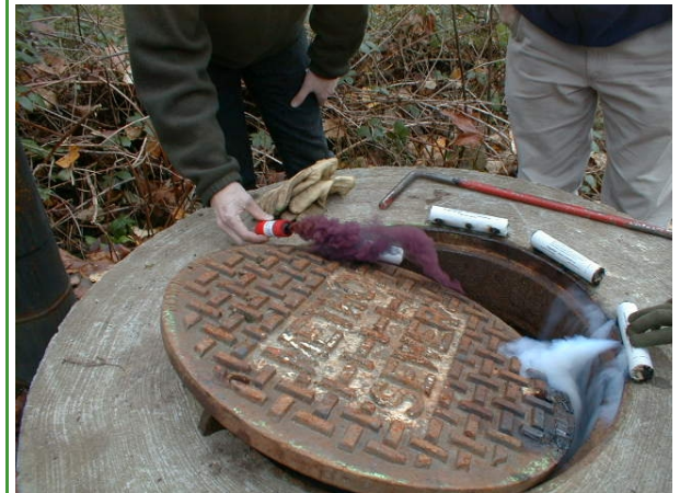
Different colored smoke candles used in a manhole (Photo Credit: Herrera).
