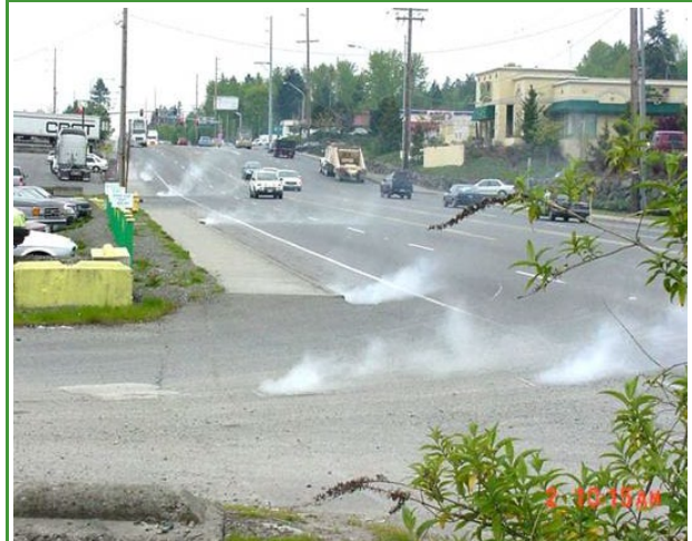
Smoke test reveals connections to the storm drainage system (Photo Credit: City of Federal Way).
