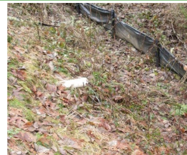
Cheater pipe (Photo Credit: Herrera).
