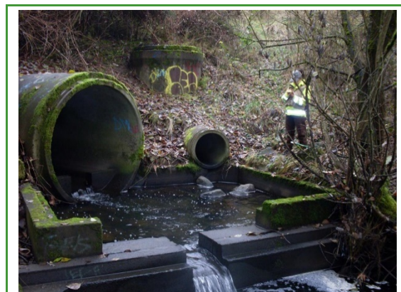
Outfall inspection (Photo Credit: Herrera).
