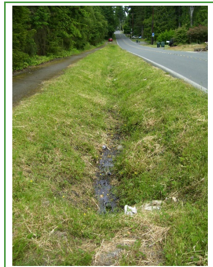
Ditch inspection (Photo Credit: Herrera).
