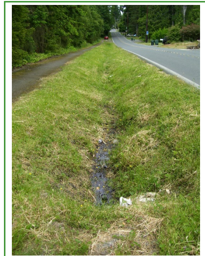
Ditch inspection (Photo Credit: Herrera).
