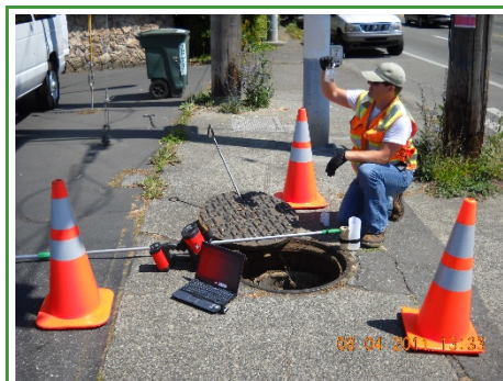
Manhole inspection (Photo Credit: City of Seattle).
