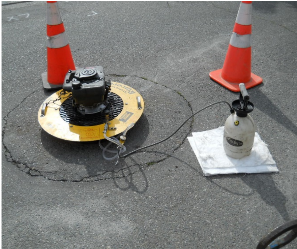
Smoke testing engine and liquid smoke in place during smoke test (Photo Credit: City of Seattle).
